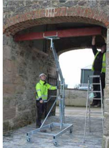
The unique beam lifter is an easy to operate lifter suitable for lifting steel, wood beams or other materials into position. Lifts up to 600kg to heights of 3m but will fold down and fit into most estate cars.
