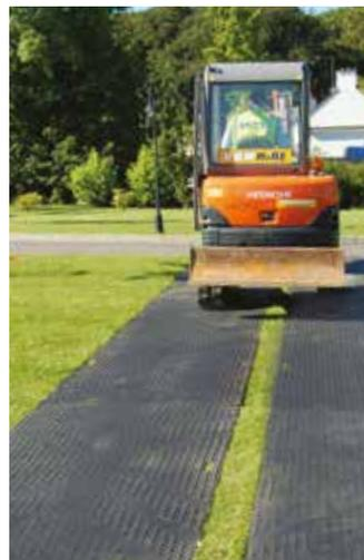
Ground Protection & Pedestrian Mats provide temporary access and ground protection for pedestrian or vehicle movement. These mats are easy to handle with pedestrian mats coloured to demarcate pathways etc. Ground mats can distribute loads of up to 60t and used as roadways or to form parking and turning areas.
