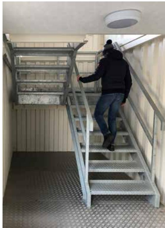
These purpose built staircase modules provide quick and easy access to stackable modular building configurations either 2 or 3 floors high. Internal and external stairway options are available and have been designed and manufactured to allow quick erection on-site, ideal for a wide range of applications on small or large construction or industrial sites.
