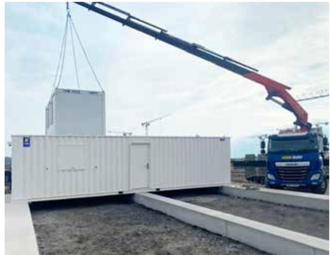
Link-Space units can be stacked side by side up to 3 storeys high with external staircases used to access the link corridor. These units offer the most cost-effective way to provide large accommodation space in a quick time frame so you can start work on-site immediately. Linked units can be configured to suit your layout requirements including offices, canteens, drying rooms and meeting rooms, along with toilets and showers.
